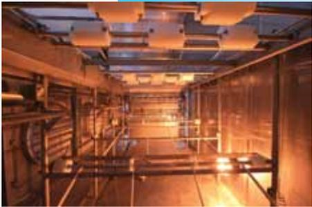
Multi-set fan section located under the conveyor belt
